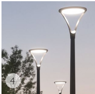
4 Replace light head fixtures
