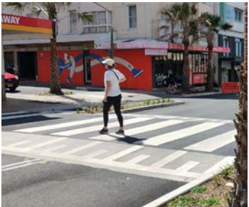
Raised pedestrian crossing
