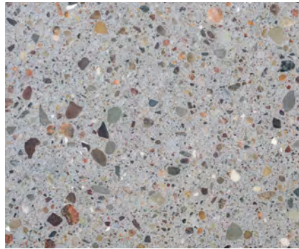
Feature concrete paving
