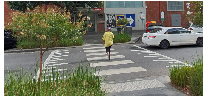
Raised pedestrian crossing example: South Melbourne
