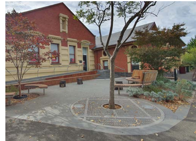
Tree grate example, South Melbourne
